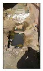
Figure 10: Poor Maintenance of Property Chamber leads to blockage at home
