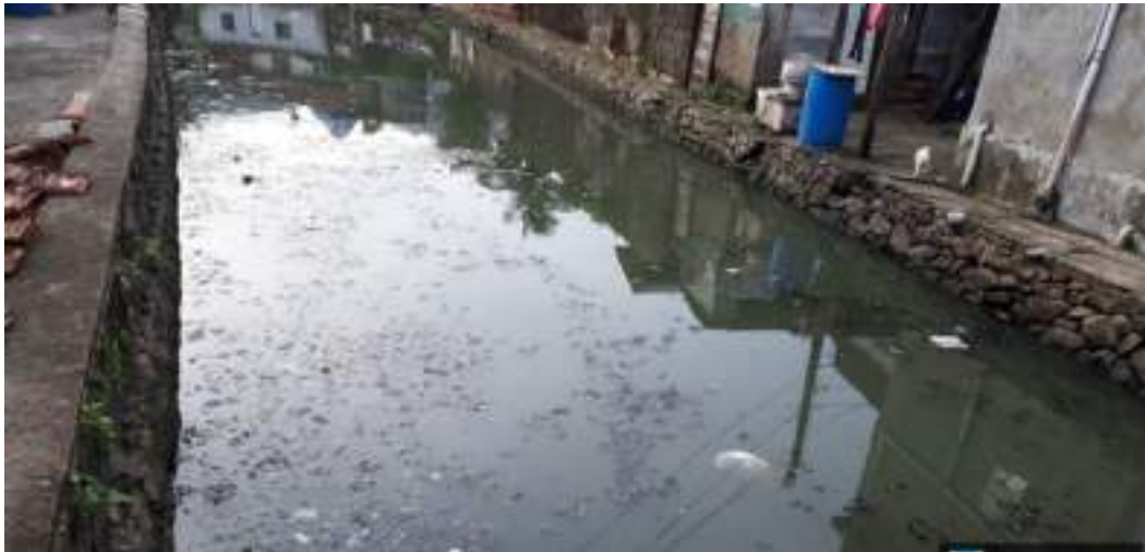
Figure 5: Direct disposal of sewage into a canal (Photo Credit: bechtel.org)
