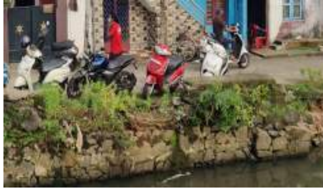
Figure 19: Relining of canals (Photo Credit: bechtel.org)
