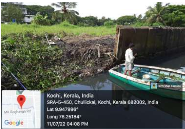
Figure 5-9 Canal cleaning activities
