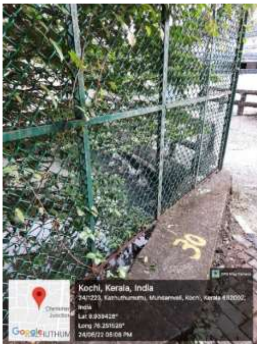
Figure 7-4: Fencing at Rameshwaram canal (Photo credit: bechtel.org)
