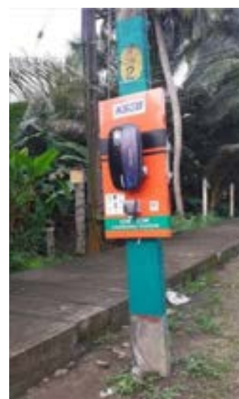
Figure 7:KSEBL Electric Pole mounted 3.3 kWh Charging Station
