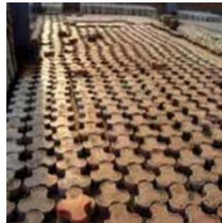
Pavers made from recycled C&D waste (Source: Bansal & Singh, 2013)
