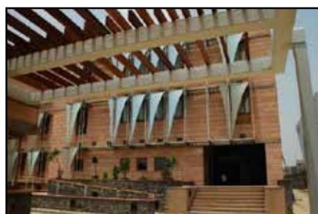
The Institute of Rural Research and Development at Gurgaon uses soil excavated from its basement to produce CSEB Blocks for its masonry and for its landscape garden slopes.
