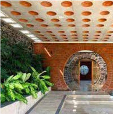
Filler slab construction (Source: Blurring Boundaries, n.d.)
