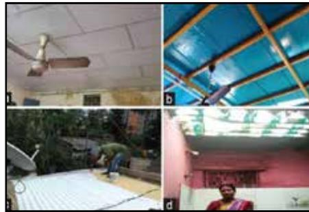
Four intervention type roofs: (clockwise) (a) Thermocol ceiling, (b) Modroof, (c) Solar reflective white paint, (d) Airlite ventilation.
