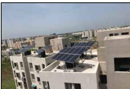
Rajkot Municipal Corporation (RMC) deployed rooftop solar PV systems in SMART GHAR scheme (social housing) to offset the energy demand of common utilities such as water pumps, elevators, common lighting.
