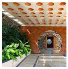
Filler slab construction (Source: Blurring Boundaries, n.d.)
