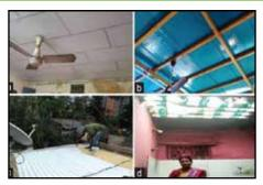
Four intervention type roofs: (clockwise) (a) Thermocol ceiling, (b) Modroof, (c) Solar reflective white paint, (d) Airlite ventilation.
