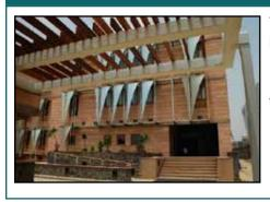
The Institute of Rural Research and Development at Gurgaon uses soil excavated from its basement to produce CSEB Blocks for its masonry and for its landscape garden slopes.
