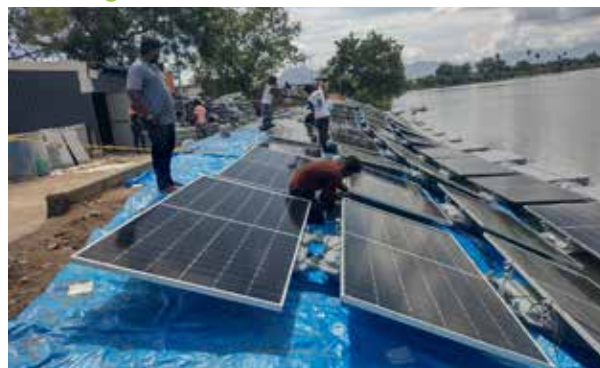
October 2024, Periyakulam Lake, Coimbatore, Tamil Nadu, India: The Coimbatore City Corporation issued a work order to ICLEI South Asia for the implementation of a 140-kWp Floating Solar PV plant at the lake, under the state's Namakku Naame scheme. The capacity of the pilot was then increased to 154 kWp to ensure policy compliance.
