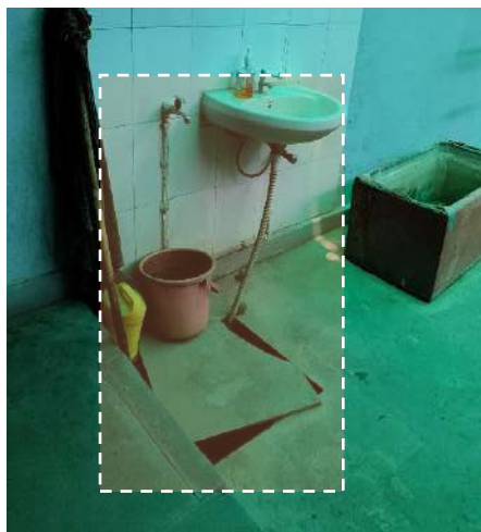
Figure 46: Handwashing station in a state of disrepair at the Sector 14 PHC. Its height is also not appropriate for small children.
