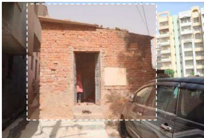
Figure 39: Poor condition of AWC in Goverdhan Vilas 2, with temporary leaky roof, and unplastered walls that invite dampness and related risks.
