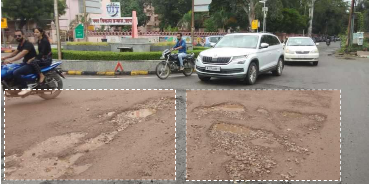
Figure 19: Poorly maintained roads and absence of lane marking (Location: UIT Circle).
