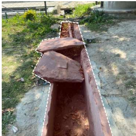
Figure 28: Open and damaged drains in Gulab Bagh, Udaipur.
