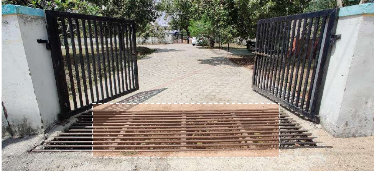
Figure 48: Cowcatcher grill at Madri PHC. which makes it unsafe for young children and stroller to pass over
