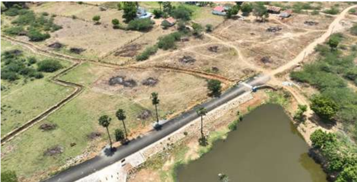
Channel and Surplus weir restored
