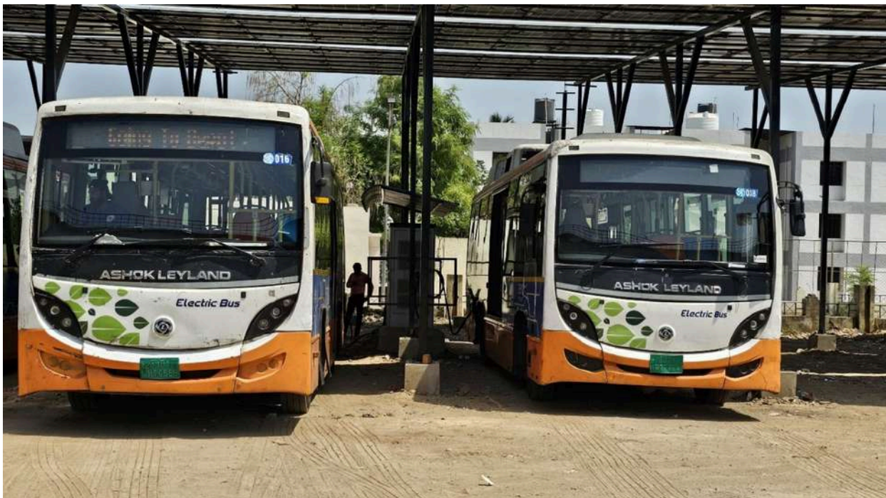
Solar Powered Opportunity Charging Depot and Electric Bus Fleet, Ahmedabad
