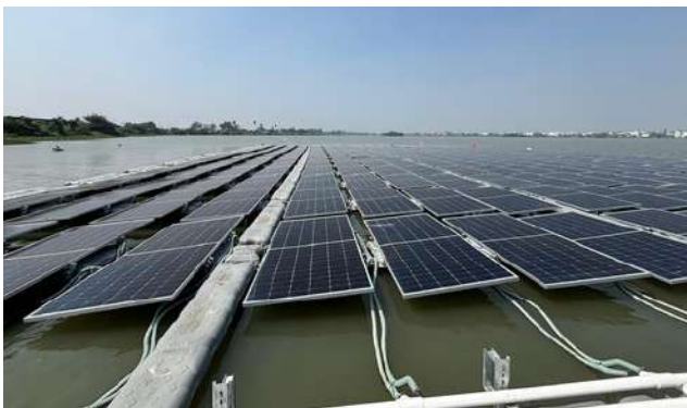
154 kWp FSPV Plant (Clockwise from top left: Site location map with HT evacuation point, aerial view of the floating solar array, inverter control room, and close-up of solar modules on floaters)
