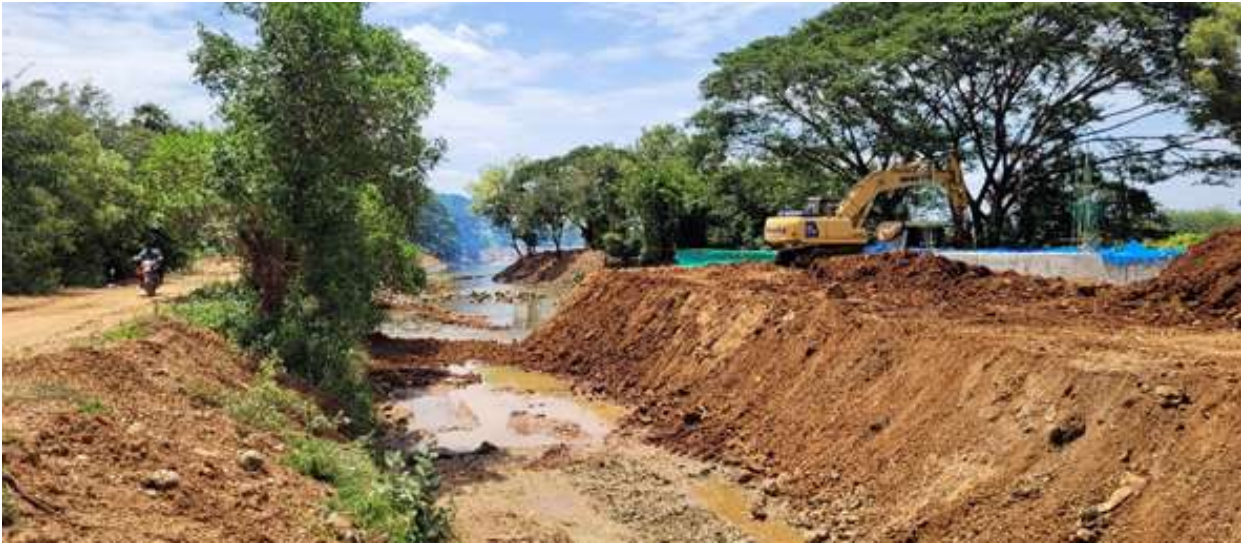
Desilting and Bund Strengthening
