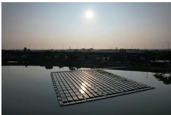
Floating Solar Photovoltaic Installation at Periyakulam Lake, Coimbatore
