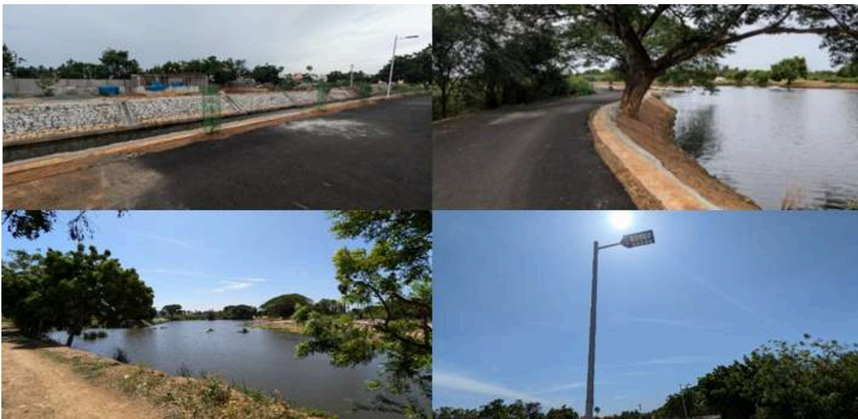
Improved surplus gate, channel, and bund with stone pitching, native tree plantation, solar-powered street lighting at Chettikulam Lake
