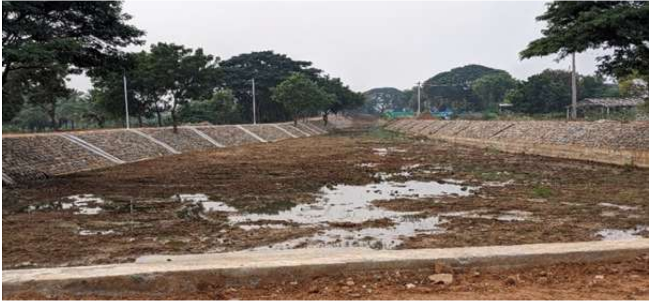
Bund Improvement work
