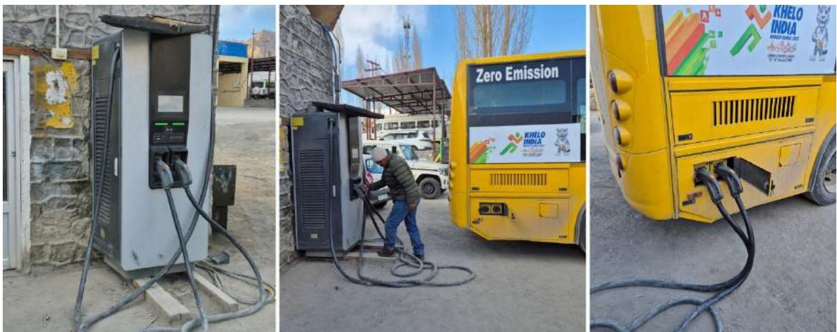
Figure 15: E- bus charging
