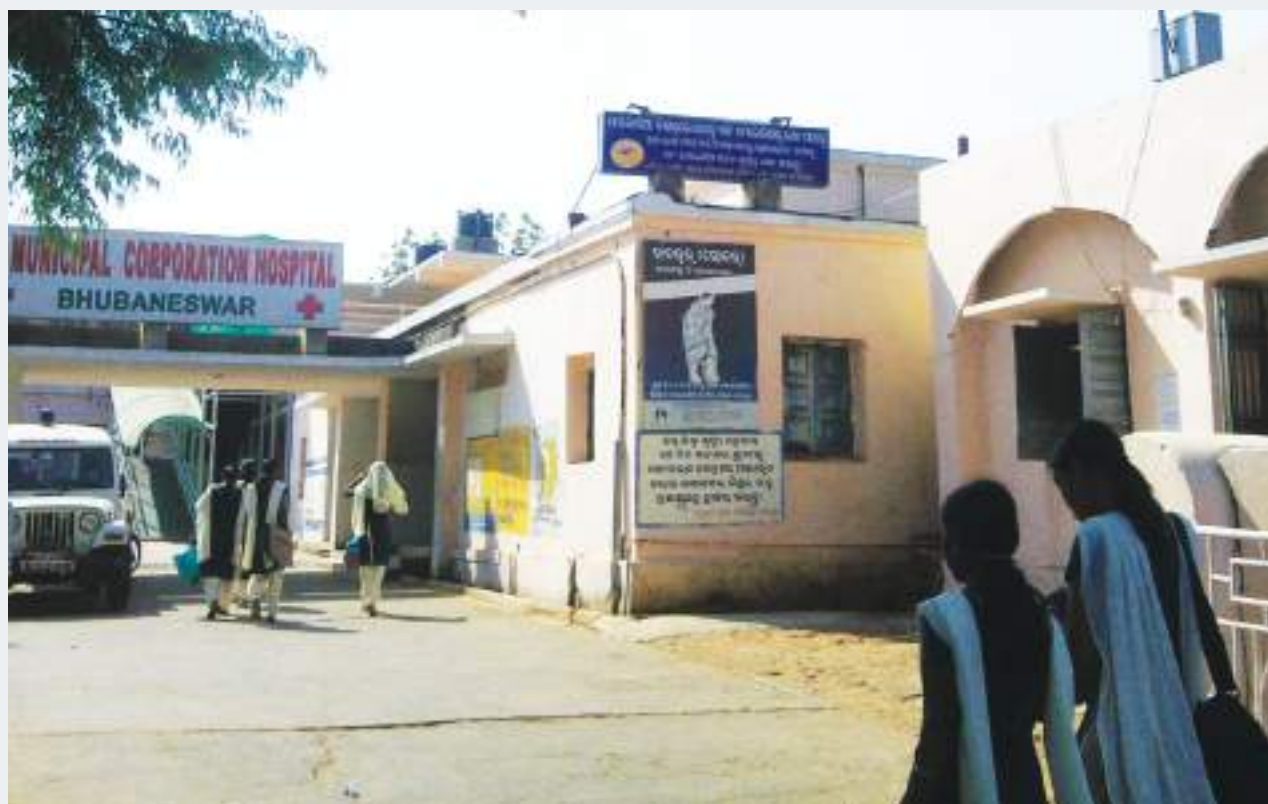
Solar PV lighting in Bhubaneswar municipal hospital, Application of RE and EE in the Urban Health Sector project, 2009
