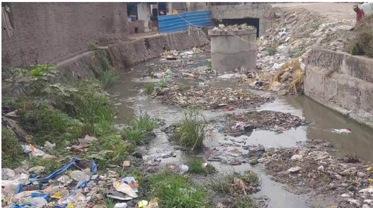
Figure 10: Kham river before restoration (Photo Credit: EcoSattva)
