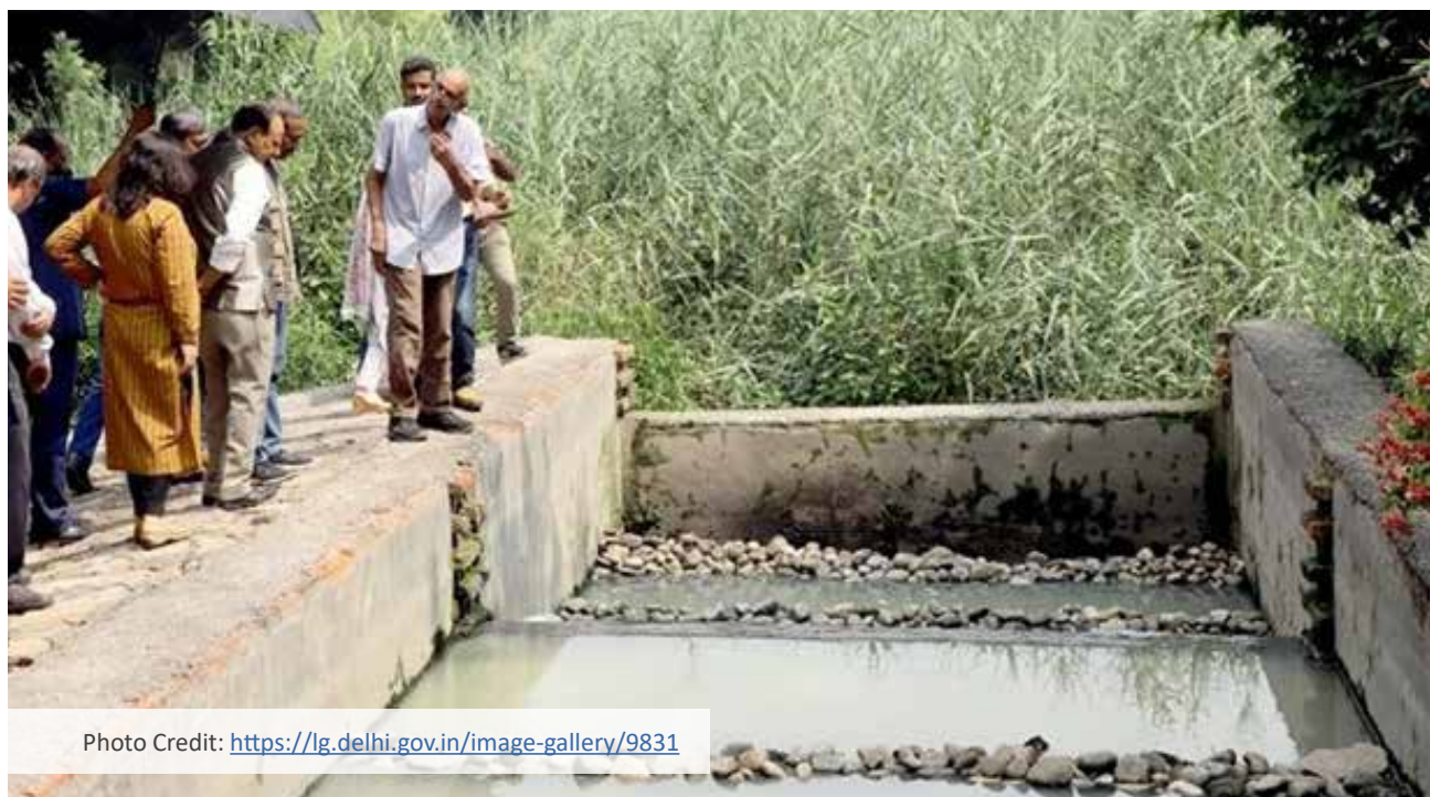
Figure 13: Constructed wetland at Neela Hauz
