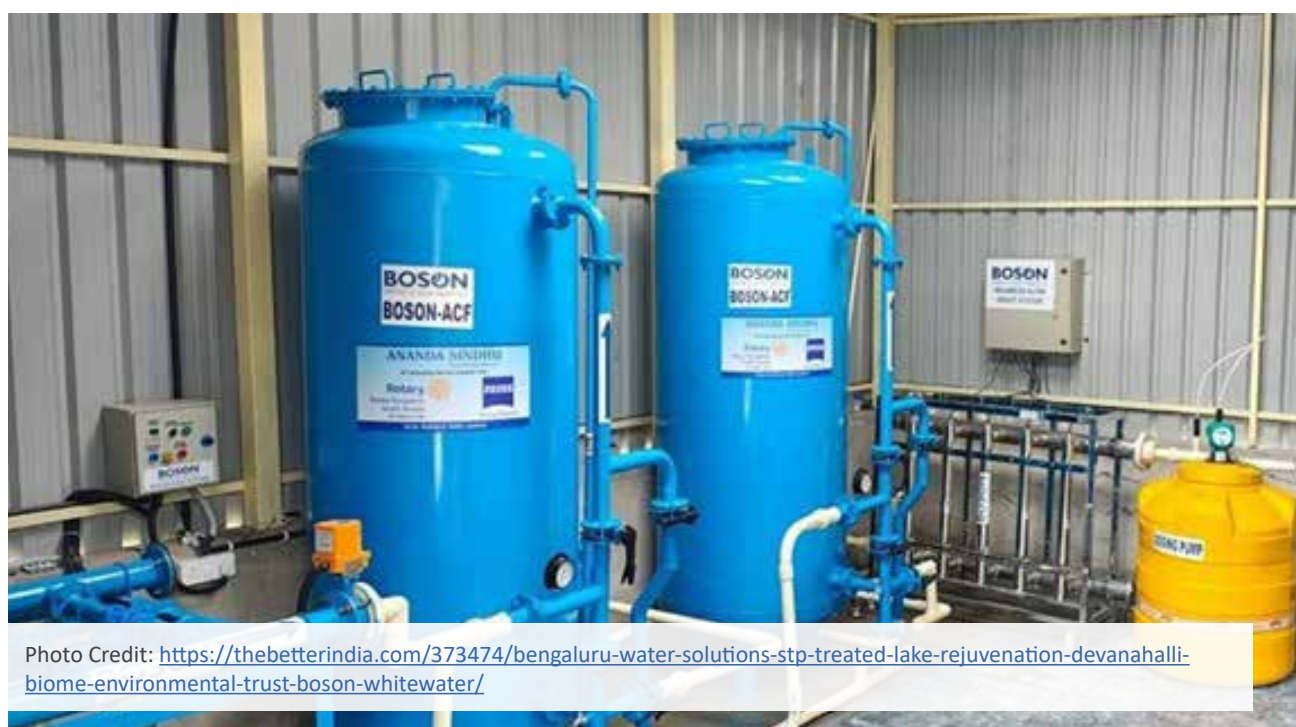
Figure 7: Tertiary treatment
