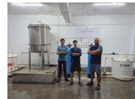
Scale-pilot validation in Bihar: 4,500 LPH design capacity and 325,731 L treated in the reported operating period
